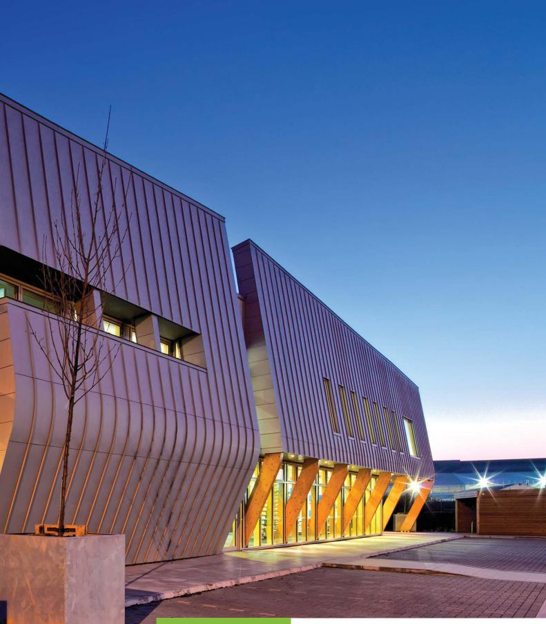
Case study | Commercia Treglown Court, Cardiff Hybrid Series 3 curtain wall Treglown Court is the new Cardiff office of Stride Treglown, the UK's 15th largest architectural practice. The building incorporates a ground level recessed front facade of Hybrid Series 3 curtain wall integrated into the glulam frame complemented by Hybrid windows. To the rear, the building features a striking timber-clad façade glazed with Senior's Hybrid windows.
